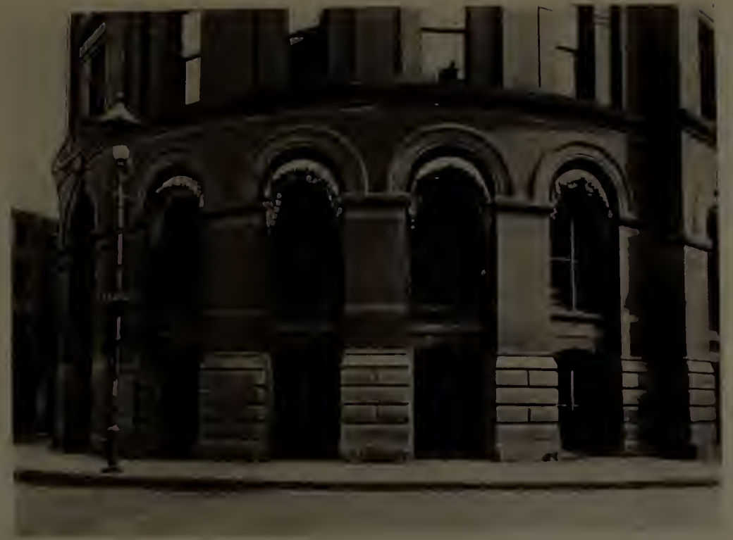
OFFICES OF THE CHINA MUTUAL INSURANCE COMPANY (Marine), Mason Building, 70 Kilby Street, Liberty Square.
